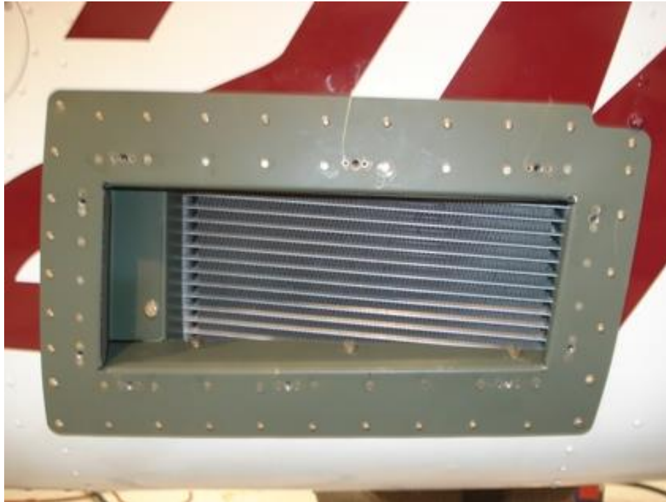
Figure 8 – External Condenser Installation
