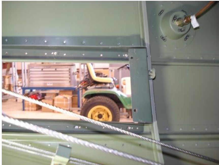
Figure 4 – Location of Outlet Flange Assembly
