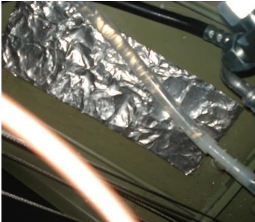
Figure 12 – Aft Evaporator Drain Line
