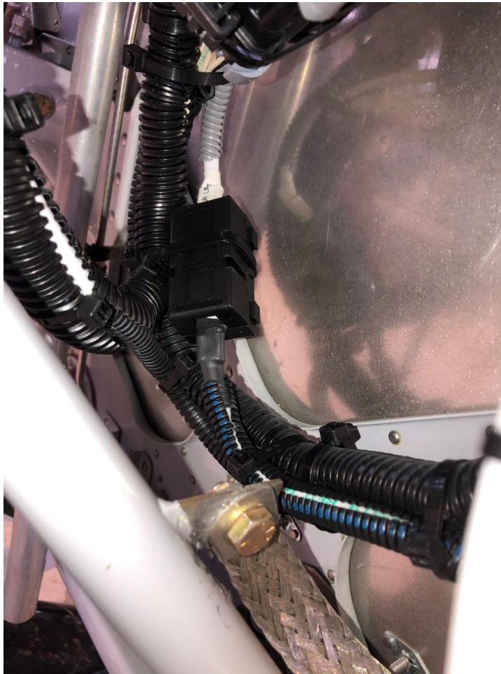
Figure 3 – Installation of 70 Amp Fuse and Fuse Holder Below J Box
